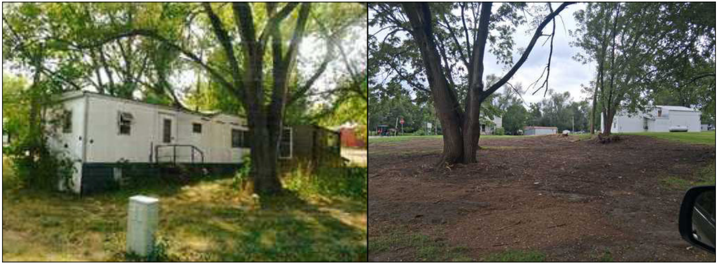
LOT CLEAN-UP. Milton Lions helped remove a dilapidated trailer house from a property in town. This included cutting down and hauling away major brush and tree overgrowth on the lot. Pictured above is the before on the left and the after on the right.
